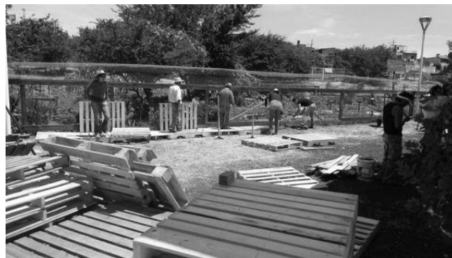
Figure 7: PAZ construction process.
